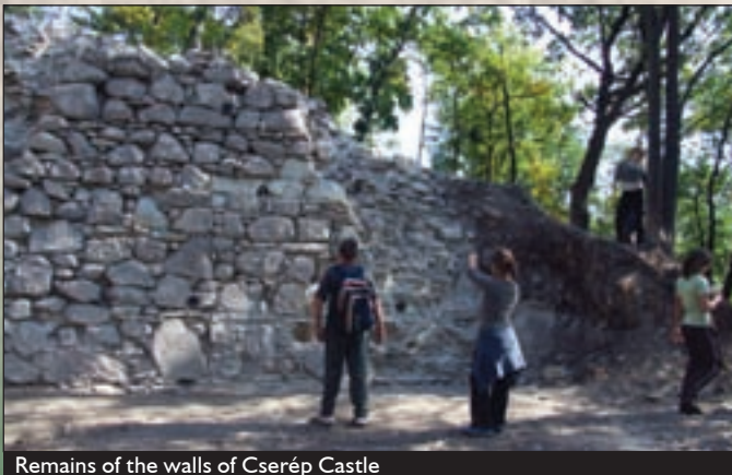
Remains of the walls of Cserép Castle
